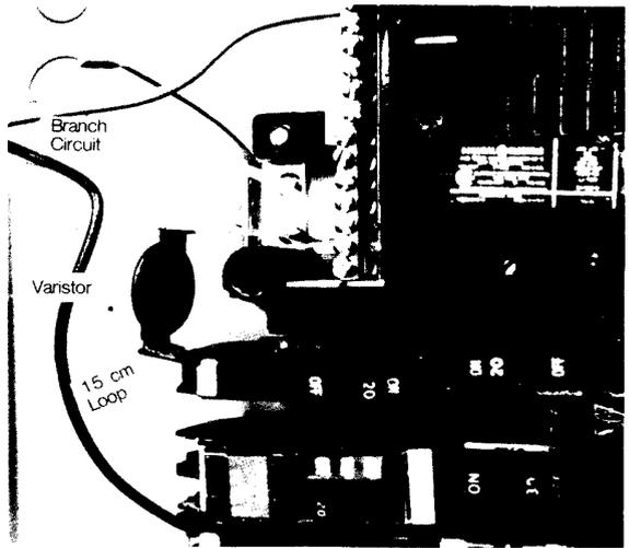
Figure 15: Installation of varistor with short connections
