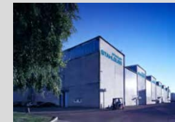
Stadler Stahlguss 120 employees
