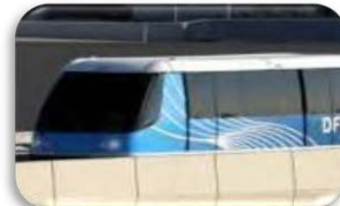
APM Systems INNOVIA - Dallas/Fort Worth Airport (USA)
