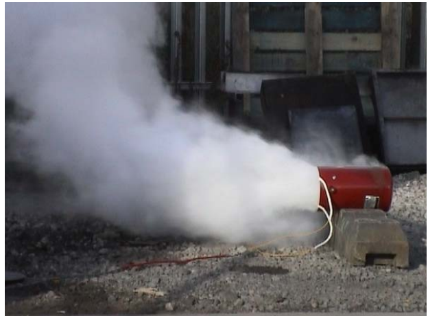
Figure 3. Discharge of a single slow discharge extinguisher unit
