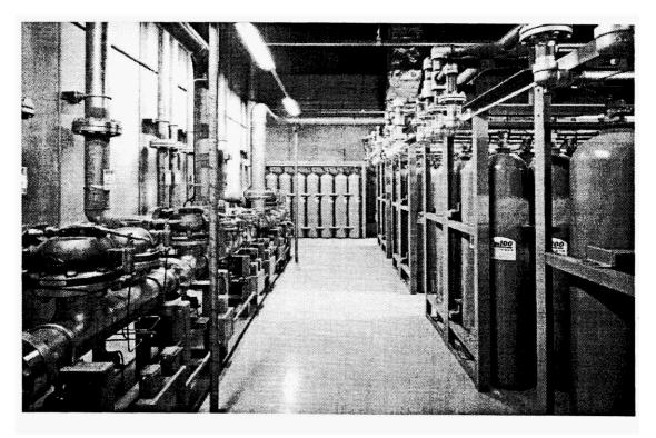
Figure 4. Typical NN100 Total-Flood Fire Suppression System Installation.
