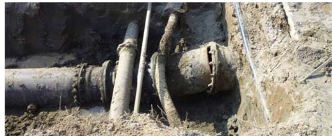
Figure 9-4. Liquefaction Caused Differential Settlement Between Pile-Supported Structures and Buried Pipe during the 2011 Tohoku Earthquake (Courtesy of Don Ballantyne)
