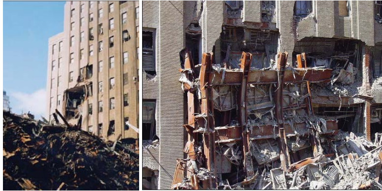
Figure 8-2. Damage to Verizon Building on September 11, 2001 (FEMA 2002)
