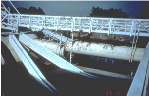
Figure 9-3. Santa Clara Valley Water District, Rinconada Water Treatment Plant Clarifier Launderers Damaged due to Sloshing, 1989 Loma Prieta Earthquake (Courtesy of Don Ballantyne)
