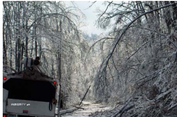
Figure 8-7. Trees Fallen Across Roads Due to Ice Storm in Kentucky Slowed Down Recovery Efforts (Kentucky Public Service Commission 2009)
