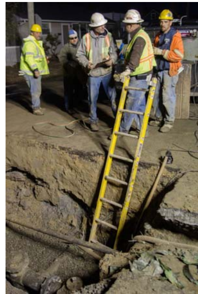
Figure 6-9: Natural gas crew shuts off gas after Hurricane Sandy (Photographer: Liz Roll, 2012)
