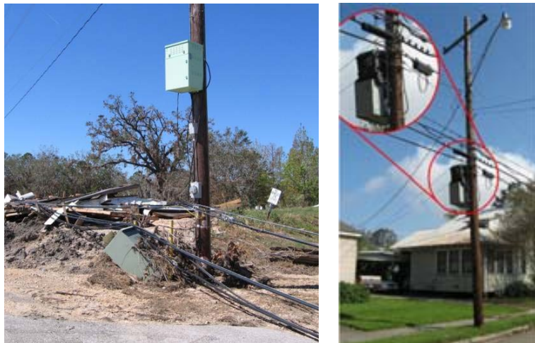
Figure 8-9. Placement of UPS Systems is an Important Consideration for Resilience and Periodic Maintenance (Kwasinski 2009)
