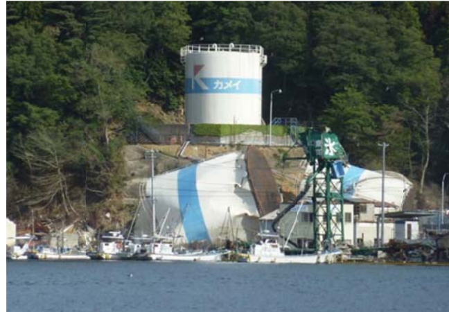
Figure 9-13: Steel Tanks Displaced Due To Tsunami Inundation, Tohoku Earthquake, Japan, 2011 (Source: Tang & Edwards, 2014)
