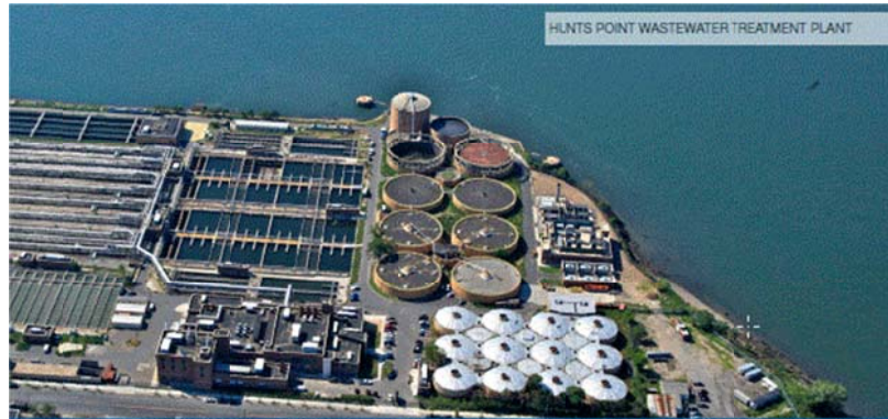
Figure 9-17: Wastewater Treatment Plants Are Often Located Adjacent To Or Along Waterways In Flood-Prone Areas. Hunts Point WWTP Along the East River In New York City Is Shown Here.
