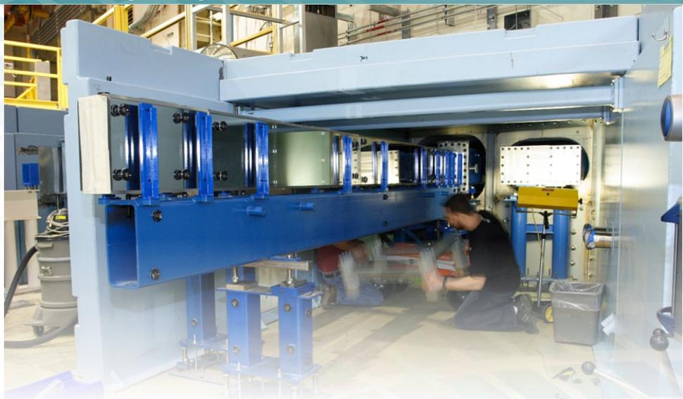
**NCNR technical staff members Dan Adler and Mike Rinehart perform installation work on the new, advanced neutron guides as part of the NCNR Expansion Project. This particular guide will provide a very high flux of neutrons for experiments performed by the Physical Measurement Laboratory Neutron Physics group**
