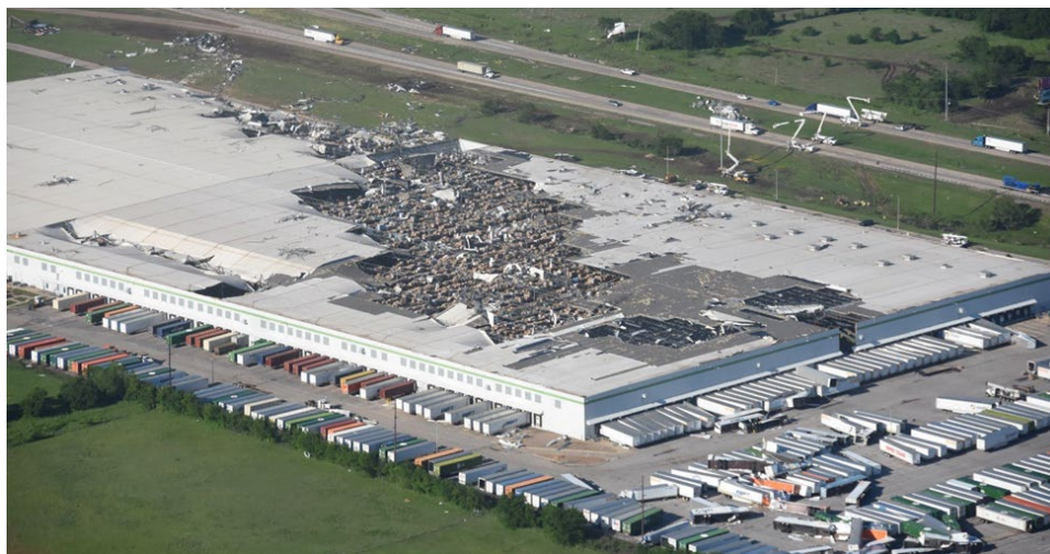
Figure 9. Tornado-damaged warehouse in Marietta Oklahoma following the April 27, 2024 storm. Source: Civil Air Patrol.
