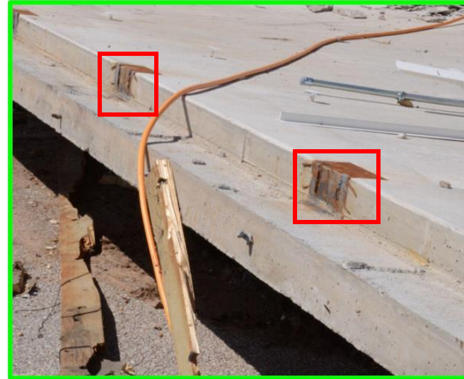
Joist Pocket; concrete wall damaged due to uplift forces
