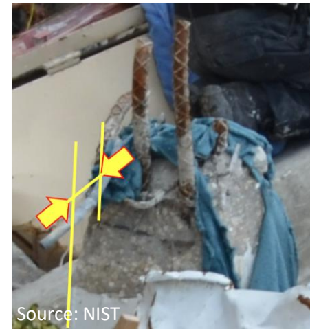
Position of Reinforcement Cage Within Columns
