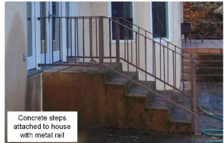
Item 32 Stairs Connected to Residence – Use a noncombustible material for exterior stairs attached to noncombustible barrier/section between steps and house (min 1') or replace with noncombustible handrail.
