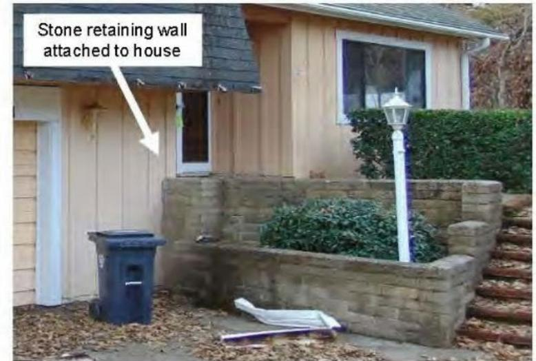
Item 34 Attached Retaining Walls – Replace retaining wall length equal to two times retaining wall height with noncombustible components.
