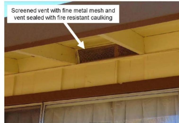
Item 14.1 Under Eave Vent (Vertical) – Keep vents clean, cover with a 1/8<sup>th</sup> inch fine metal mesh screen, and seal vent with fire-resistant caulking.
