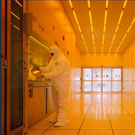
NIST Nanofabrication Facility
