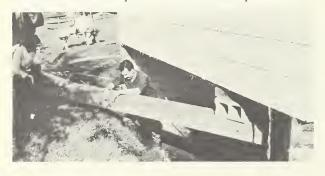
A flood in Fairbanks, Alaska in August 1967 caused extensive damage in hundreds of homes by washing out and dislocating foundations and soaking the structure and furnishings up to midheight of the first story. A visiting team of NBS engineers made recommendations that facilitated drying of the homes for early rehabilitation with a minimum removal of water-soaked building materials.
