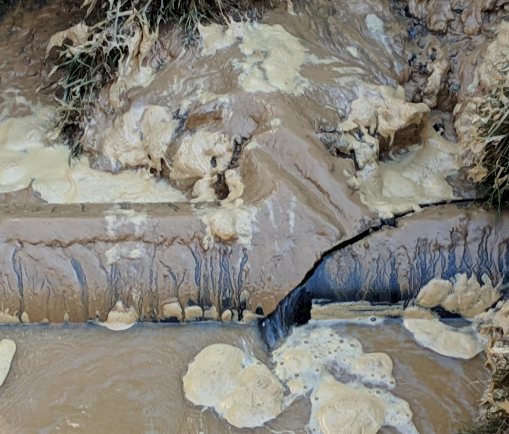
A close-up shot of a water main break at 4 a.m. on October 31, 2018. The water main break resulted in having to stop most research activities in four lab buildings for five days.
