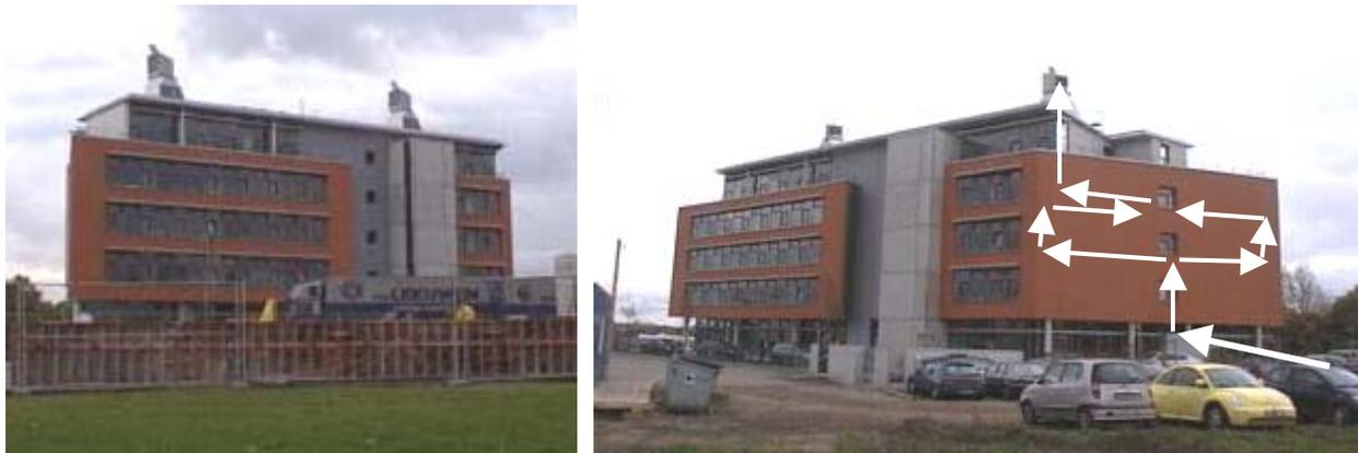
**Figure 3.12** The Gross Gerau building designed by Transsolar Energietechnik, GmbH with two dominant stacks fitted with large self-venting cowls. White arrows indicate, schematically, the ventilation airflow paths.
