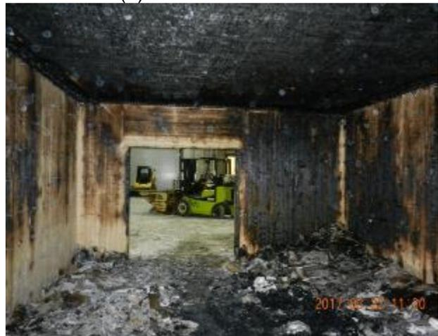
(d) interior with gypsum board removed
