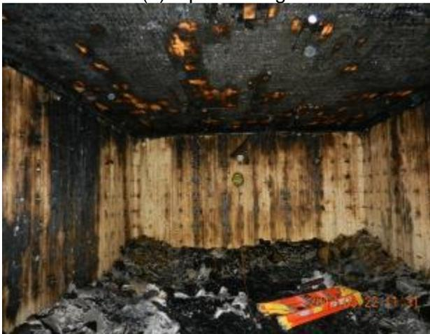
(c) interior with gypsum board removed
