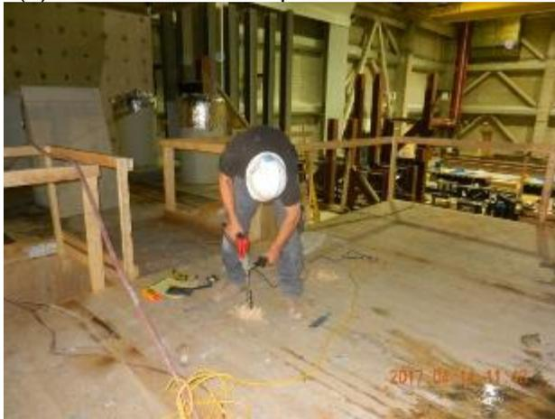
(c) drilling holes through ceiling panels
