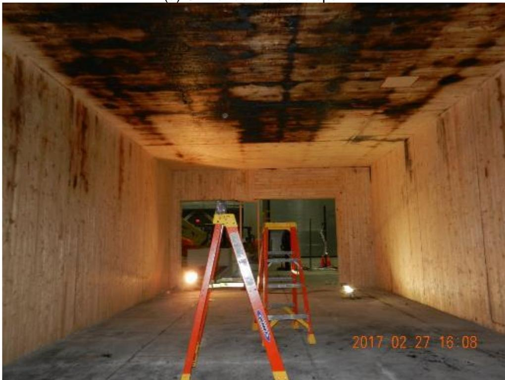
(b) CLT structure after repair
