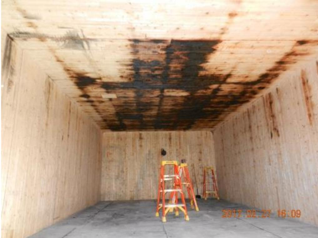
(a) CLT structure after repair
