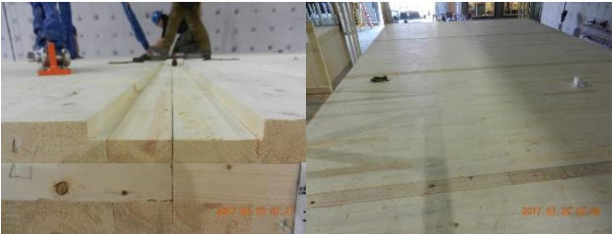
**Figure 7. Ceiling panels connected with spline joints.**
