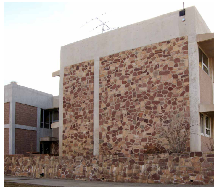
Exhibit 101: Typical Campus Lyons Sandstone Façade Materials
