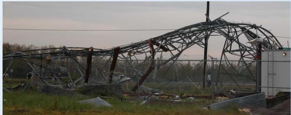
Photo credit: NIST Orange cell tower failure
