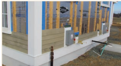
PHOTO 5 (LEFT) Cladding Attachment. Pretty straightforward. Cladding is installed over the 1 × 4 furring. PHOTO 6 (RIGHT) Done Deal. NIST Net Zero Energy Residential Test Facility, Gaithersburg, Md.
