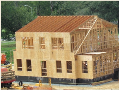
PHOTO 1 (LEFT) No Overhangs. Not yet anyway. Framing is 2 × 6 at 24 in. (610 mm) o.c., advanced framing sheathed with plywood structural sheathing. Could have been OSB. PHOTO 2 (RIGHT) Darth Vader House: Wrapped in a back fully adhered membrane. This membrane is the water control layer, the air control layer and the vapor control layer. It is clearly continuous. It is mastic sealed to the exterior face of the perimeter concrete foundation wall. We end up with an airtight concrete box at the bottom of the house (the basement floor slab is sealed to the perimeter concrete foundation wall that is sealed to a membrane wrapped sheathed structural frame. It does not get tighter than this. In terms of airtightness, it is so simple, so straightforward, so effective even a caveman can do it. Don't like black? Use a blue membrane. Don't like vapor closed? Use vapor open; it does not matter. The plywood or the OSB is the vapor "throttle."
