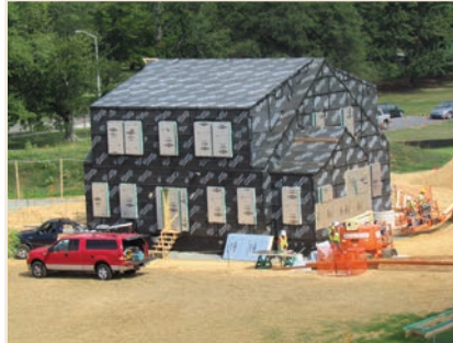
PHOTO 1 (LEFT) No Overhangs. Not yet anyway. Framing is 2 × 6 at 24 in. (610 mm) o.c., advanced framing sheathed with plywood structural sheathing. Could have been OSB. PHOTO 2 (RIGHT) Darth Vader House: Wrapped in a back fully adhered membrane. This membrane is the water control layer, the air control layer and the vapor control layer. It is clearly continuous. It is mastic sealed to the exterior face of the perimeter concrete foundation wall. We end up with an airtight concrete box at the bottom of the house (the basement floor slab is sealed to the perimeter concrete foundation wall that is sealed to a membrane wrapped sheathed structural frame. It does not get tighter than this. In terms of airtightness, it is so simple, so straightforward, so effective even a caveman can do it. Don't like black? Use a blue membrane. Don't like vapor closed? Use vapor open; it does not matter. The plywood or the OSB is the vapor "throttle."
