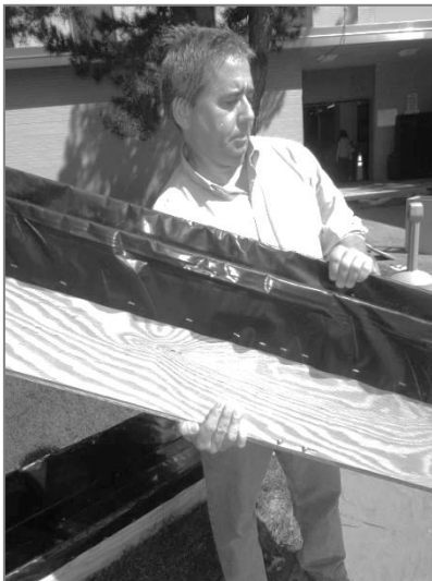
Exhibit 9. Showing how to hold a chute for the pour.
