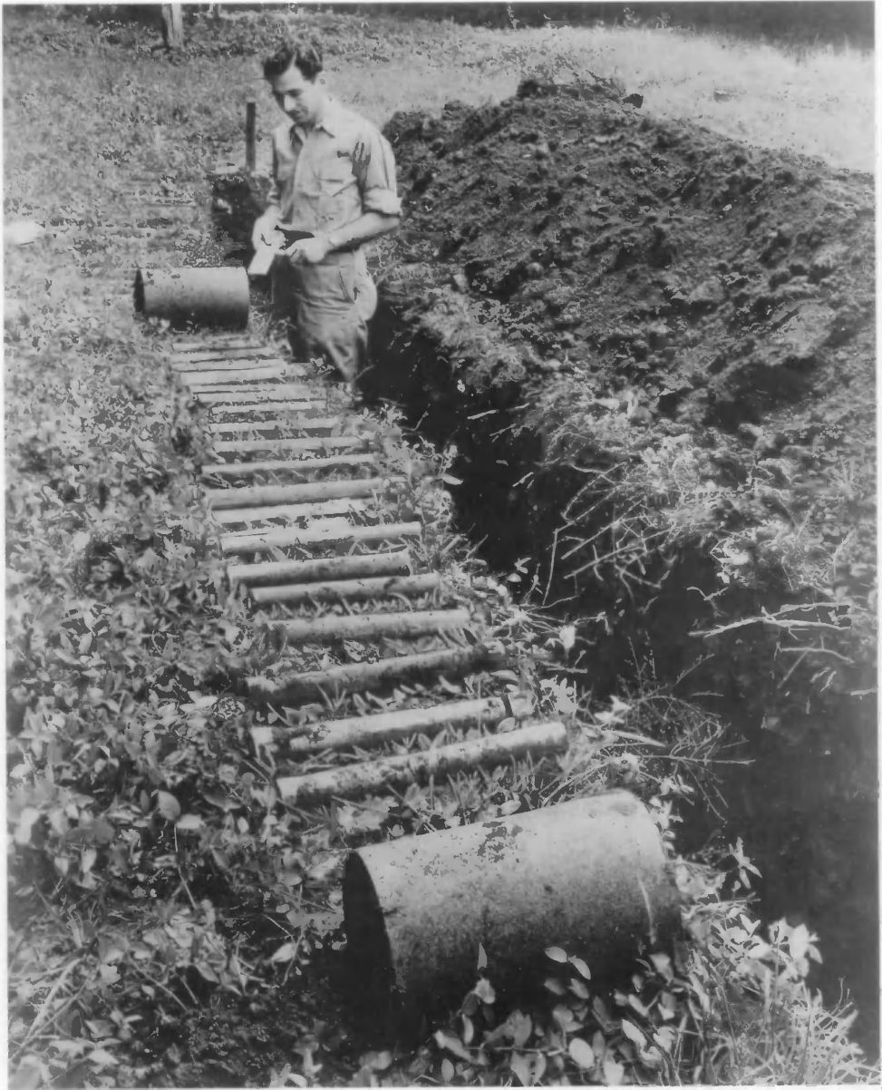
In 1949, Melvin Romanoff of the NBS Corrosion Section removed and inspected test specimens at a corrosion test site at Loch Raven, Maryland. Romanoff, an internationally known expert on underground corrosion, joined NBS in 1937; except for a year's military service during World War II, he worked at the Bureau until his death in 1970.
