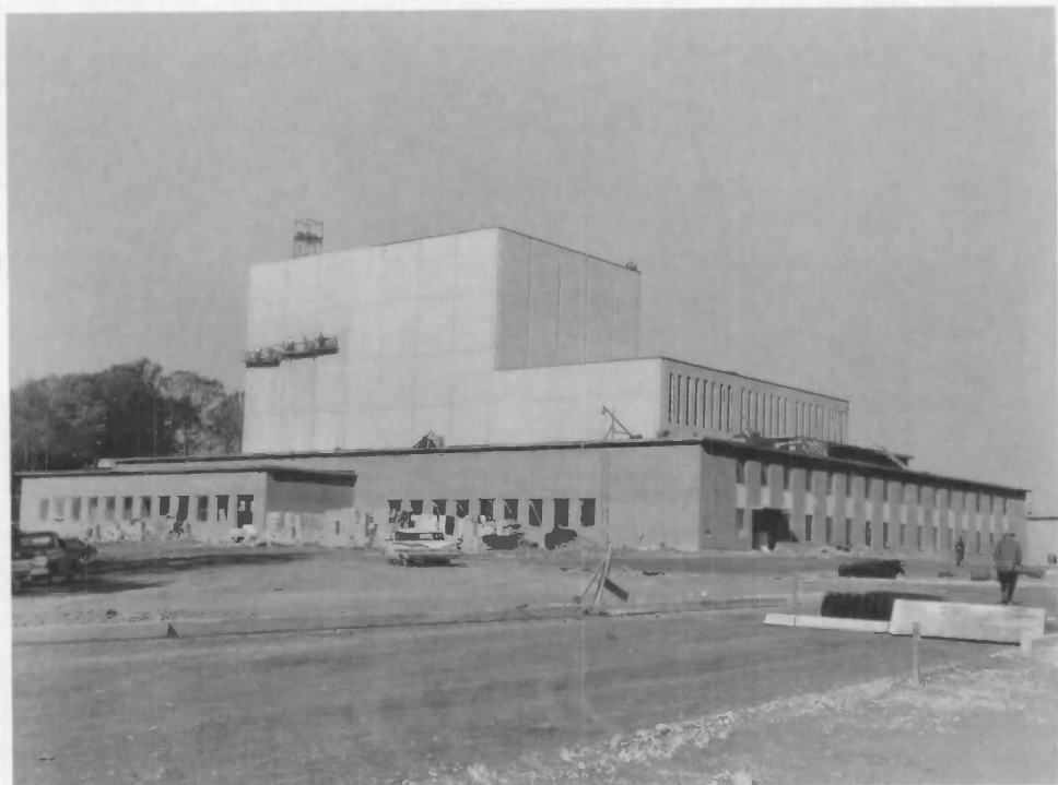
The National Bureau of Standards Engineering Mechanics Building in Gaithersburg, Maryland. It was built to house a one-million-pound dead-weight tester.
