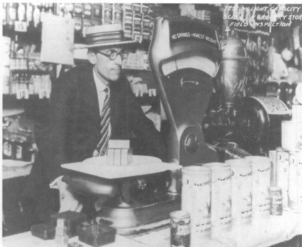
A Baltimore city inspector tested a grocery store scale for accuracy, about 1920. Photo appears courtesy of the Maryland Department of Agriculture (Weights and Measures Section).
