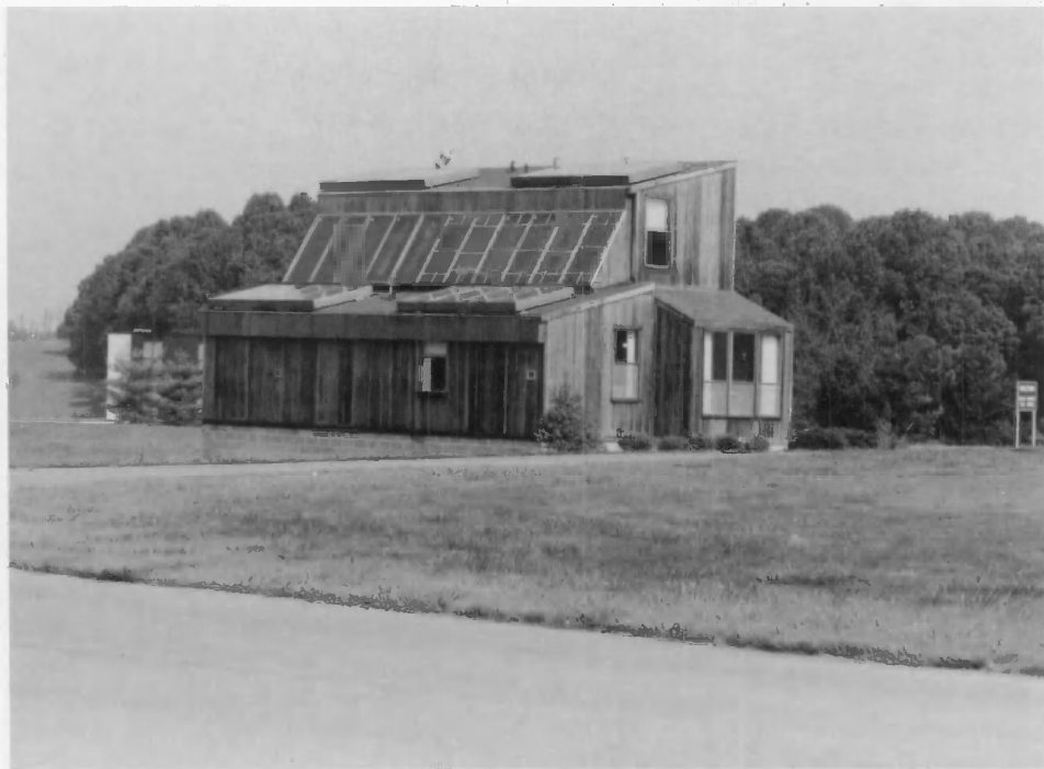
Solar collectors were installed in the National Bureau of Standards solar townhouse, a laboratory for a number of energy-conservation studies.
