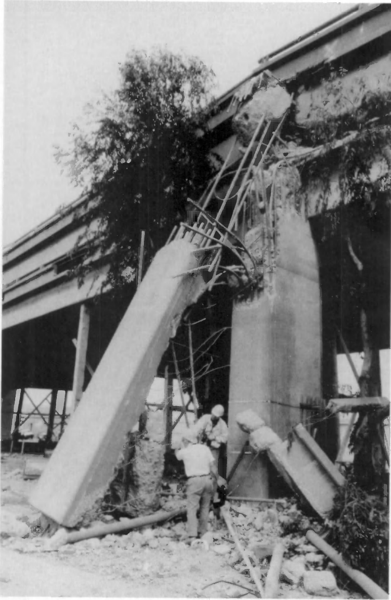
NIST Structures Division engineers H. S. Lew and Nicholas J. Carino investigated structural damage to the two-tiered Nimitz Freeway, which collapsed during the 1989 Loma Prieta Earthquake.
