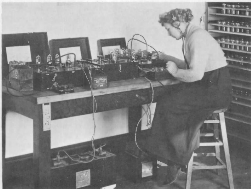
The use of the three-electrode (triode) electron tube was practically unknown to our military forces prior to 1917, and all of their apparatus was of the damped-wave type. The Bureau began testing electron tubes, as shown here, a month after we entered the war, and reported testing 467 of them up to mid-1919.
