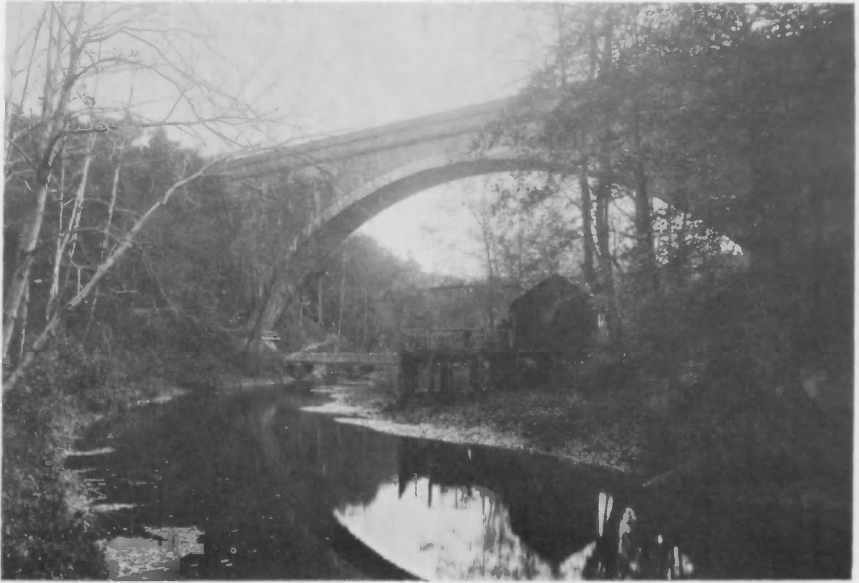
Still the largest stone arch in America, the Cabin John Bridge was completed in 1859, a 220-foot span carrying a water conduit and carriage way over Cabin John Creek. For 44 years it was the largest masonry arch in the world, until larger ones were built in Saxony and France. Since then masonry has been replaced by concrete in great bridges, as more economical.
