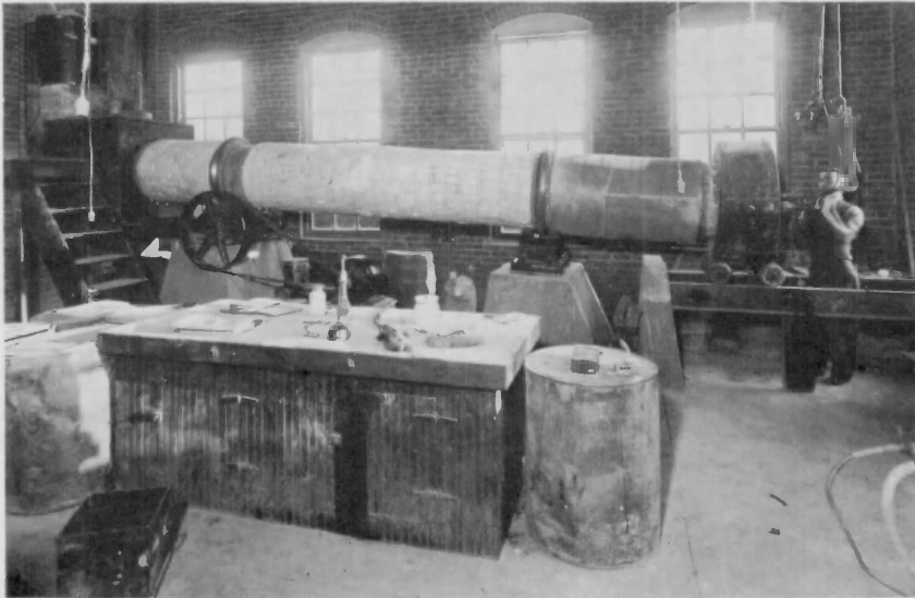
Above, the NBS small-scale experimental paper mill in which all the operations of paper-making could be studied under controlled conditions. Below, the rotary cement kiln at the Pittsburgh laboratory, brought to Washington in 1918, for determining the effects of various processes in the manufacture of cements.
