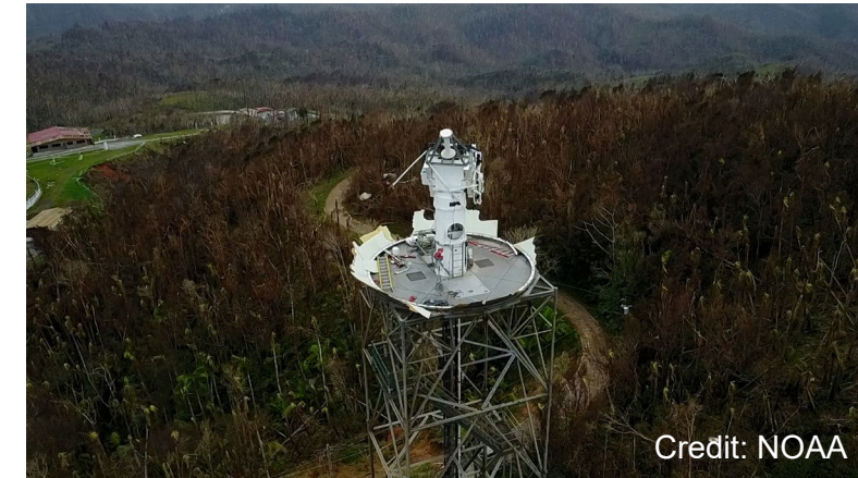
Failure of Doppler weather radar
