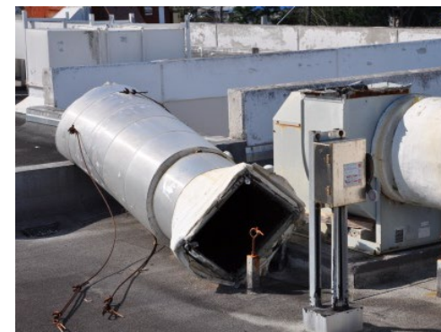
Damaged/Dislodged Rooftop Equipment
