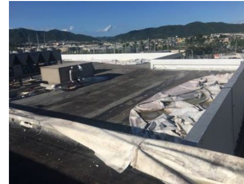
Damaged Roof Covering
