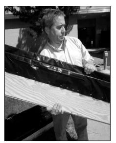
Figure 3-21. How to Hold a Chute for the Pour.
