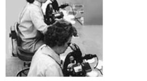
FIGURE 1. Wafer Inspection in the nineteen-sixties at Fairchild Semiconductor. Note that clean room attire was limited to a smock. Hair nets would be added by the seventies.
