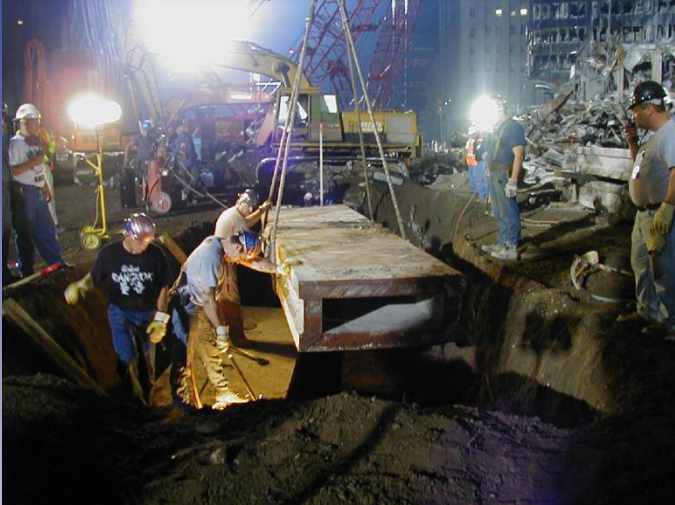
Clean weld fracture of Interior columns
