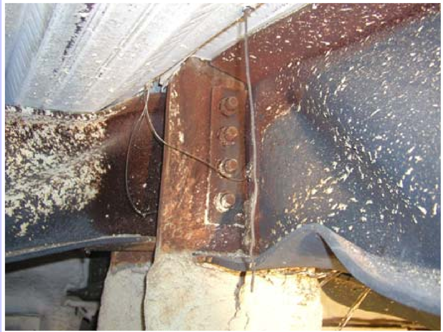
Beam shear buckling
