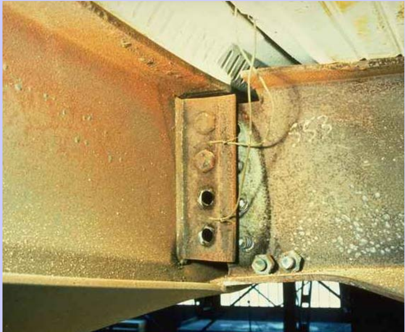
Shear failure of bolts in fin plate connection
