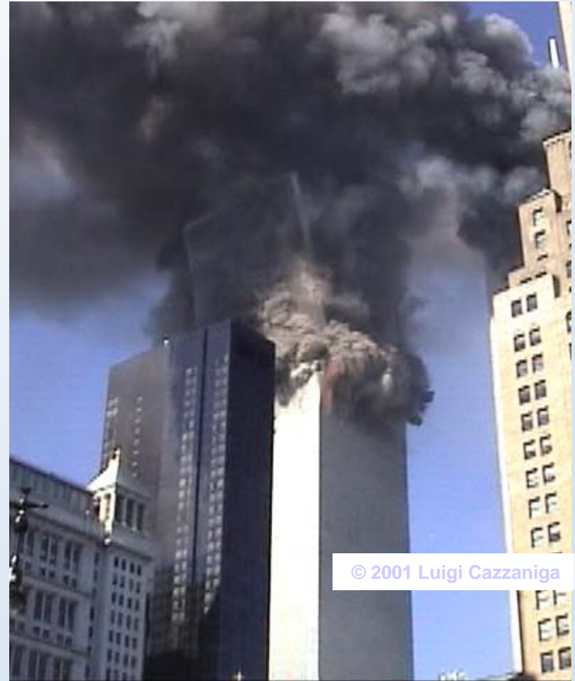
WTC 2 tilted to the east and south in this view from the northeast.
