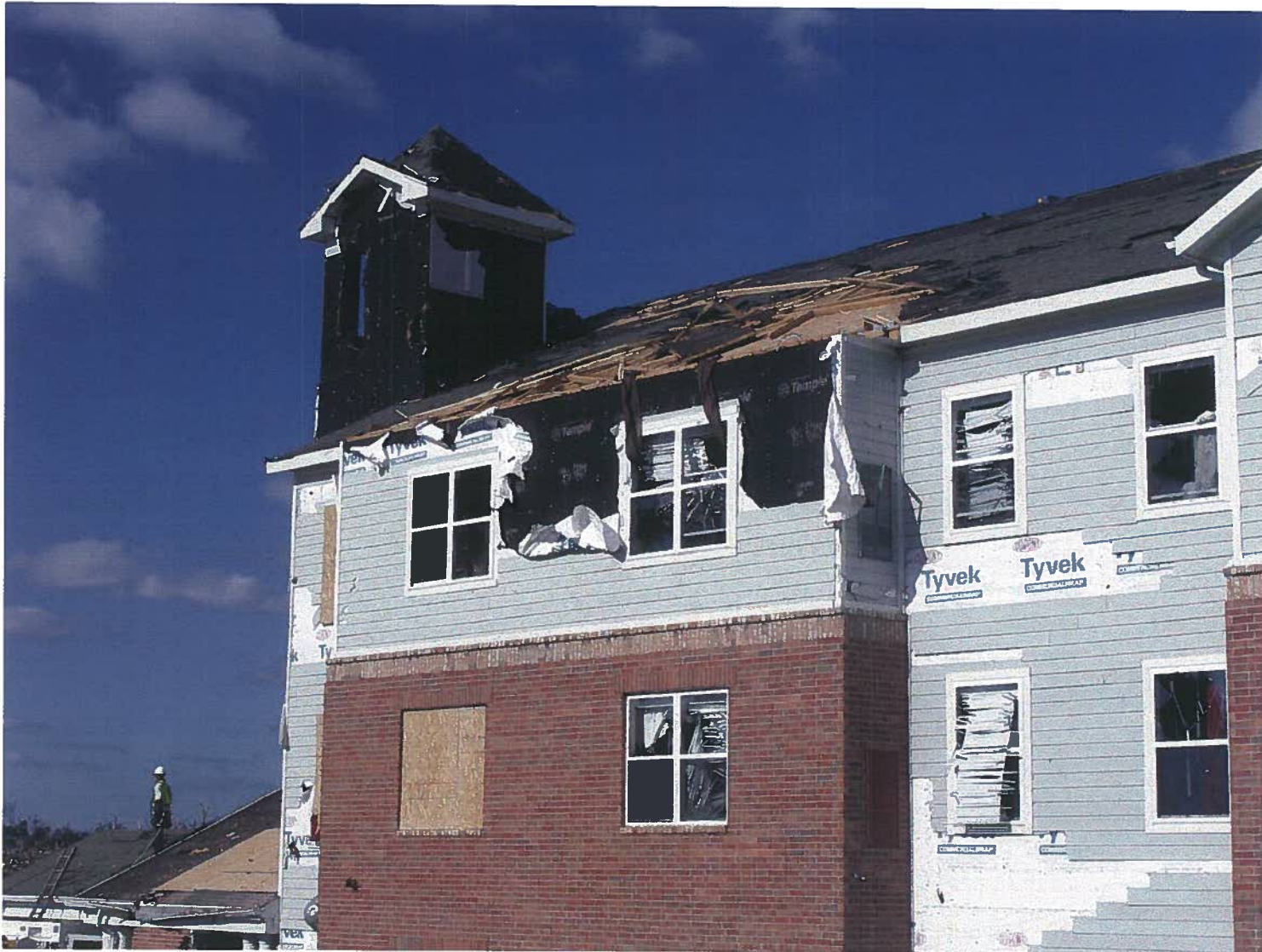
SAVE Photo 1 – Northwest corner looking northeast
