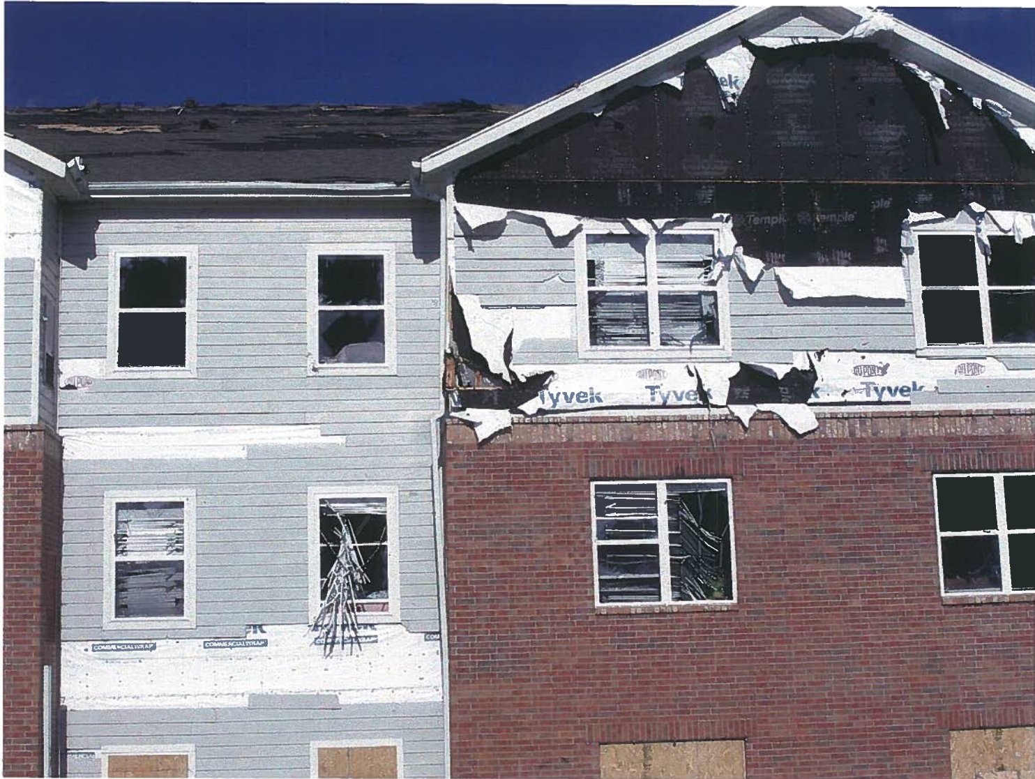
SAVE Photo 2 – West Wall, south end looking east
