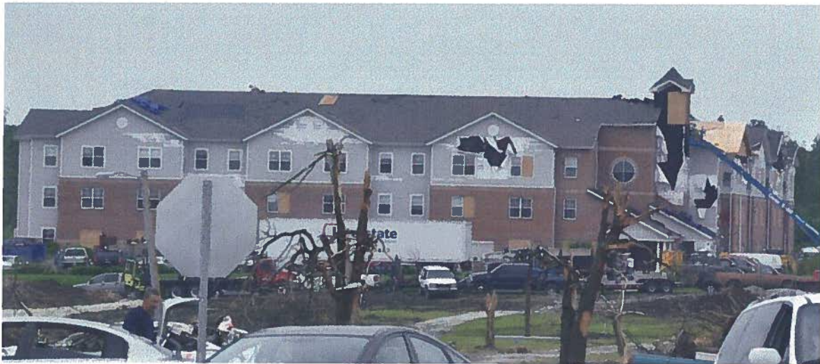
Figure 3–111. Mercy Village Apartments, viewed from the north, with envelope damage (siding, window glazing, roof covering).
