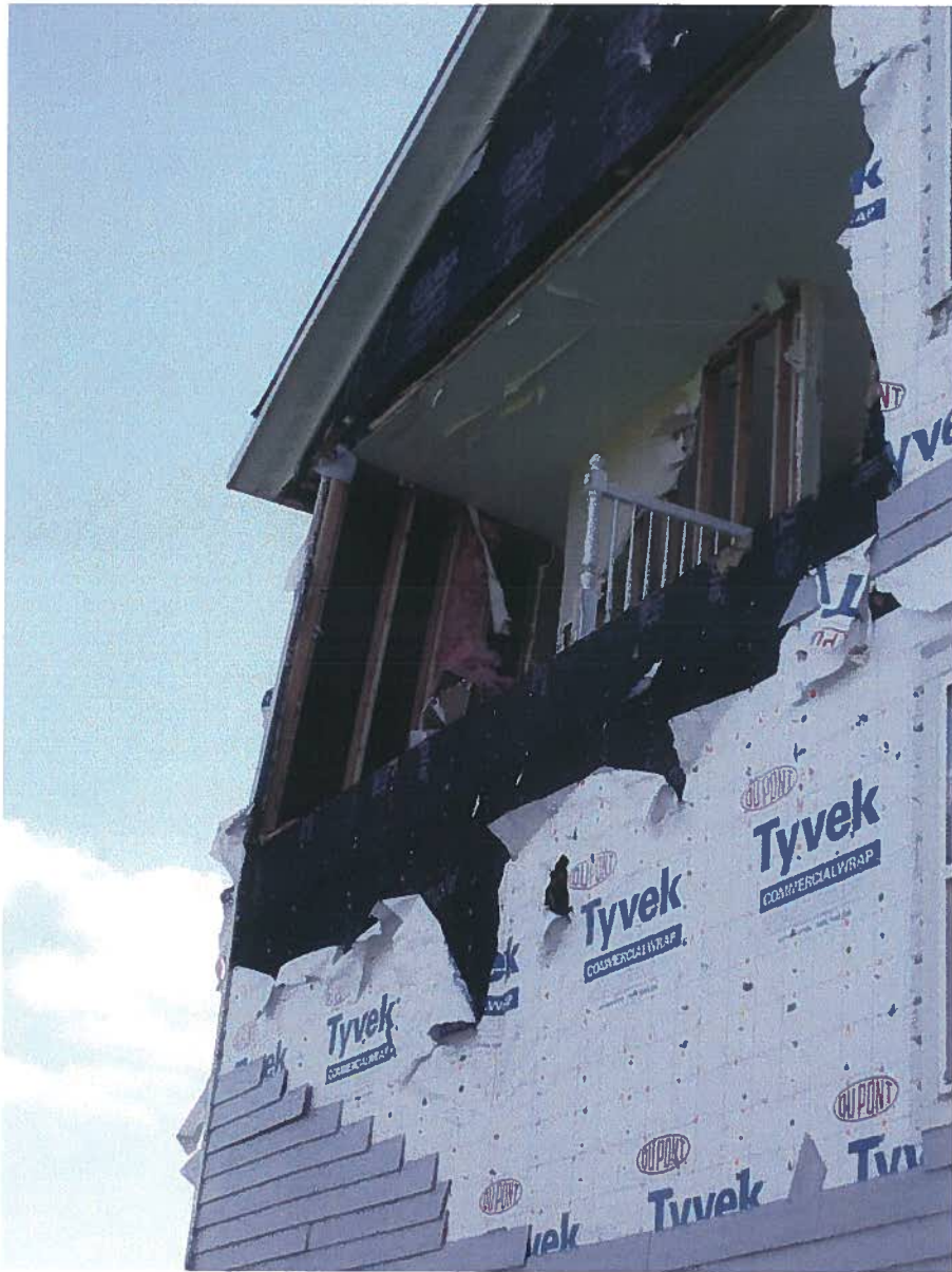
SAVE Photo 4 – East Wall, East Wing (looking northwest)
