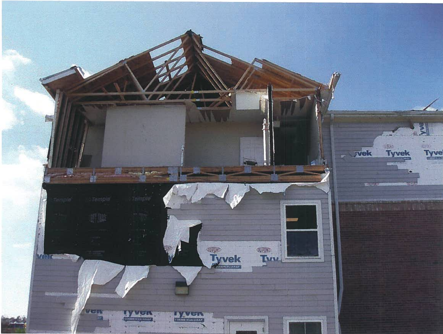
SAVE Photo 3 – South Wall, South Wing (looking north)
