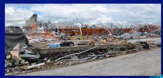
• F11: Collapses of BTS buildings typically began with failure of the roof system due to wind uplift (failure of roof *deck-to-joist* or *joist-to-wall* connections), which led to the loss of lateral bracing for perimeter walls, causing them to collapse by rotation at the base due to lateral load.
