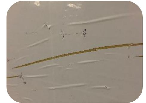
*new cracks, severe delamination and blistering*
