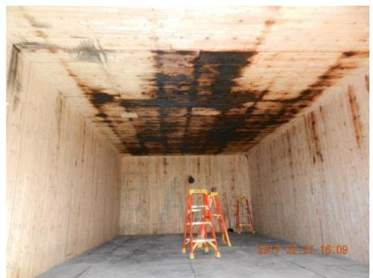
(a) CLT structure after repair
