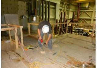
(c) drilling holes through ceiling panels
