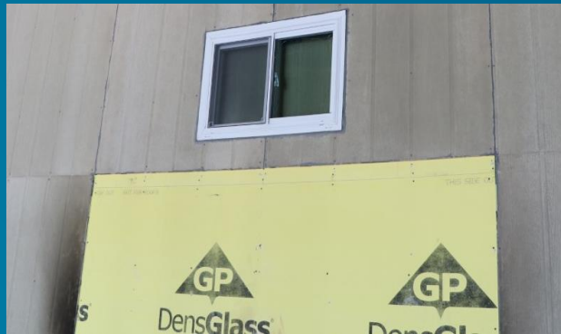
No thermal damage to sheathing
