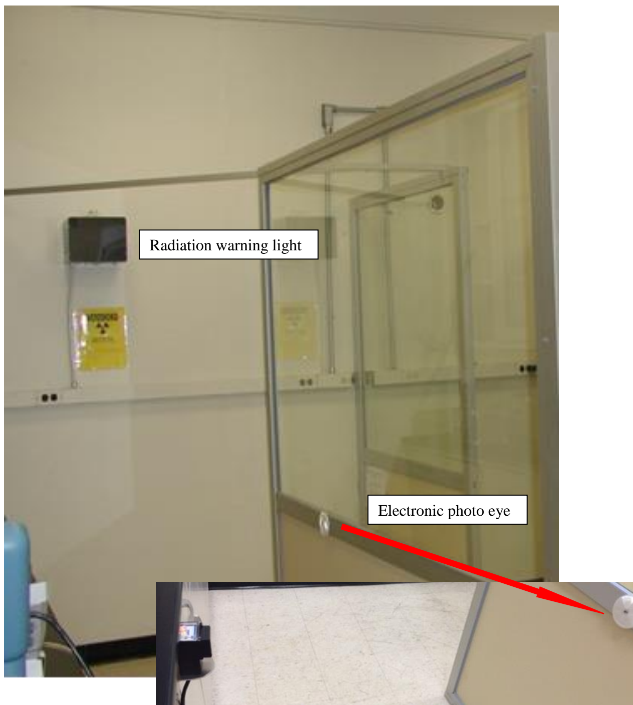
Figure 15. Two radiation safety interlocks.
