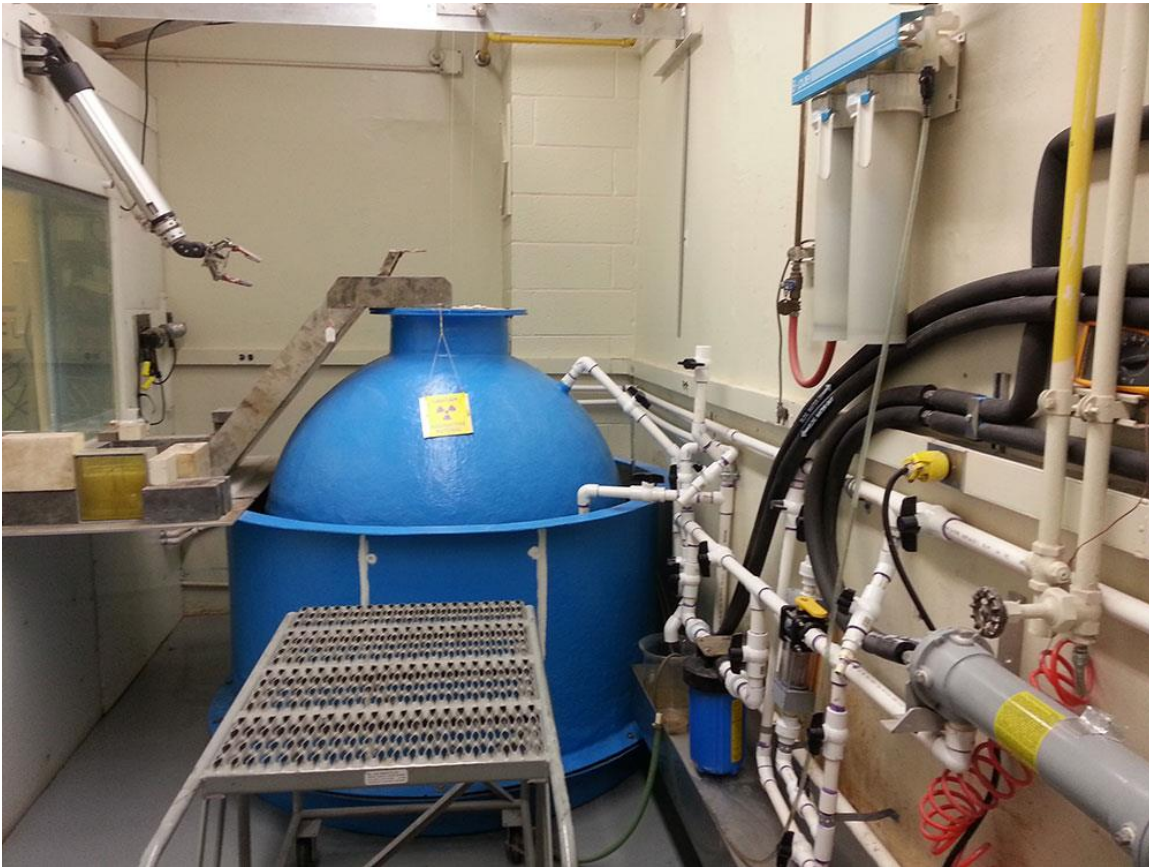
Figure 1: The manganese sulfate bath room.
