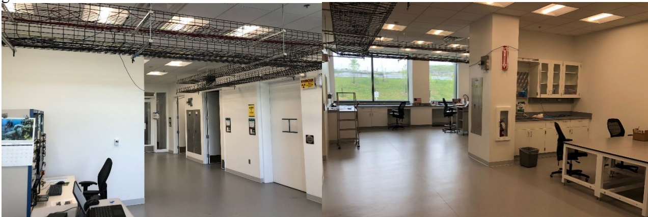
Figure 6 X-ray facility control area
