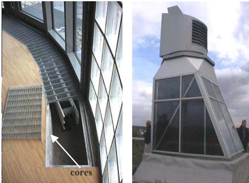
**Figure 3.13** Air diffuser detail of the Gross Gerau building designed by Transsolar Energietechnik, GmbH showing one of the cores used to direct ventilation airflows to the building perimeter. Stack terminal unit showing glazed solar assist panels and self-vaning cowl.
