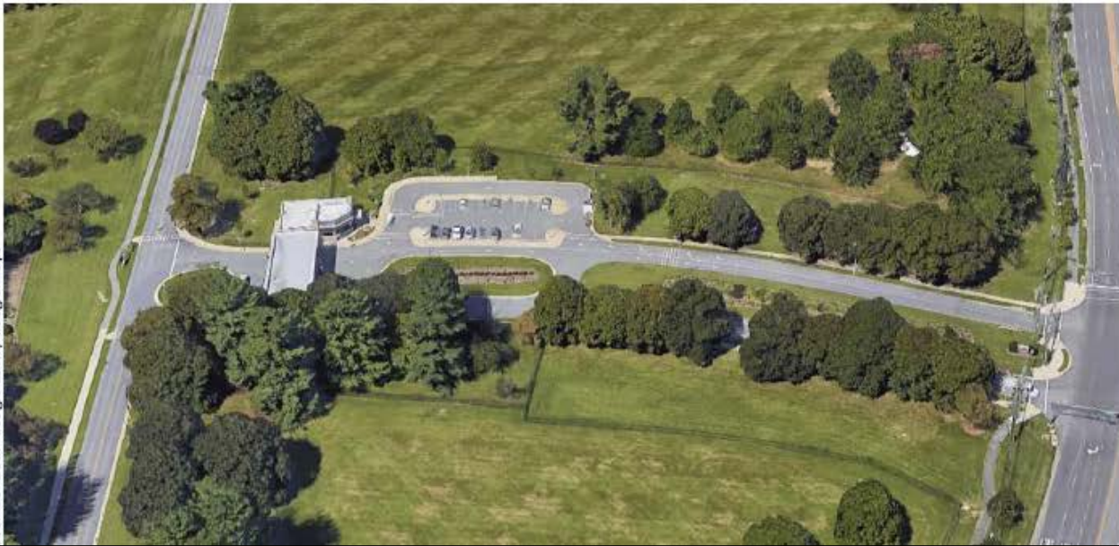
Exhibit 55: Existing Gate A Conditions
