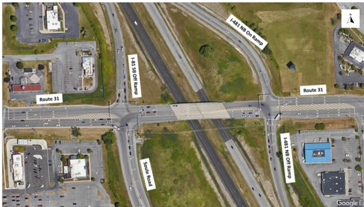
Figure 5: Existing NY 481 & NY 31 Interchange
