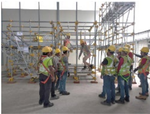
Figure 1 Work-at-Height Training scaffolding module with access and working platform for Working at Height and Rescue training and exercise.
