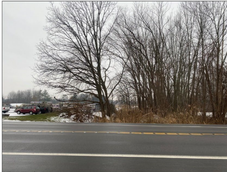
Existing view of 8642 Brewerton Road - a residence eligible for listing on the State/National Register of Historic Places
