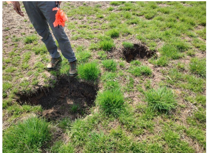
W-17 (Vertical holes show buried drainage structures are present.)
