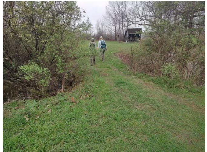
R-3 (showing the culvert to remove and ditch to fill)
