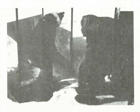
FIGURE 163 Volumetric snowpit in Ontario with sidewalls erected prior to the snow season.
