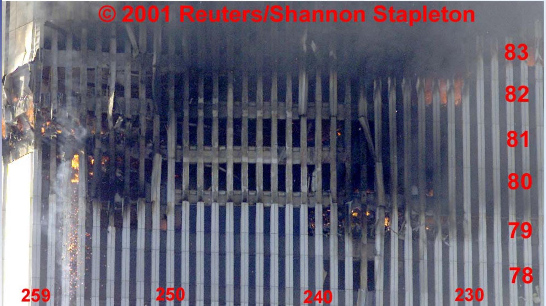
North Face of the South Tower. Image shows what appear to be portions of several floor slabs hanging across window openings on Floors 80, 81, and 82
