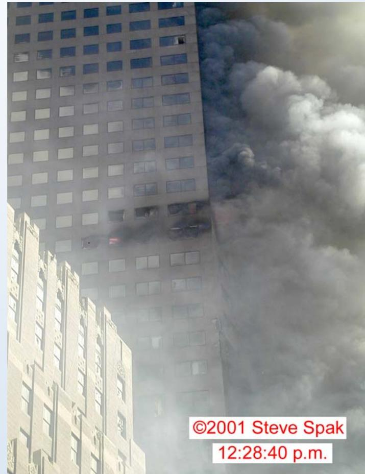
Fires in WTC 7—which began soon after WTC 1 collapsed—were observed on Floors 7, 8, 9, and 11 near the middle about half an hour before collapse; Floor 12 was burned out by this time. Fires were also seen on Floors 12, 13, 22, 29, and 30 at various times during the day.
