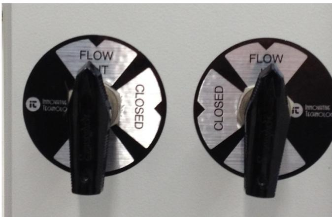
Figure 47 Oxygen analyzer valves – “Flow Out” position
