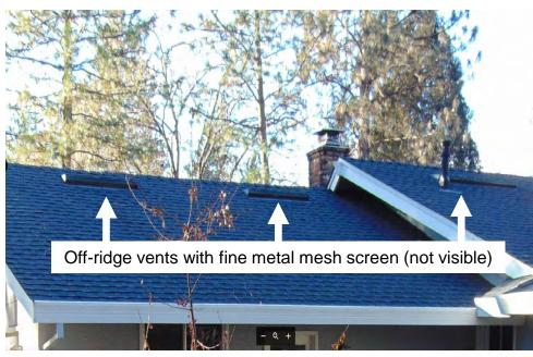
Item 12 Off-Ridge Vents – Apply fine metal mesh screens to roof vents to prevent ember intrusion.
