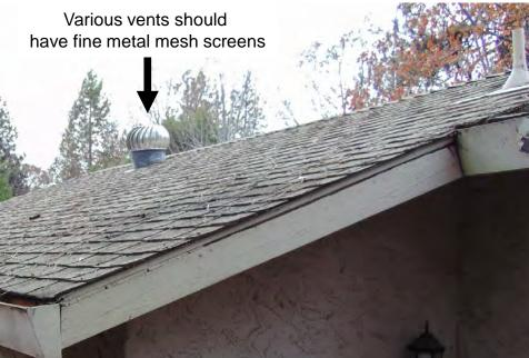
Item 17 Makeup Air Intake – Large intake vents should have a 1/8<sup>th</sup> inch fine wire mesh screen to prevent ember intrusion.
