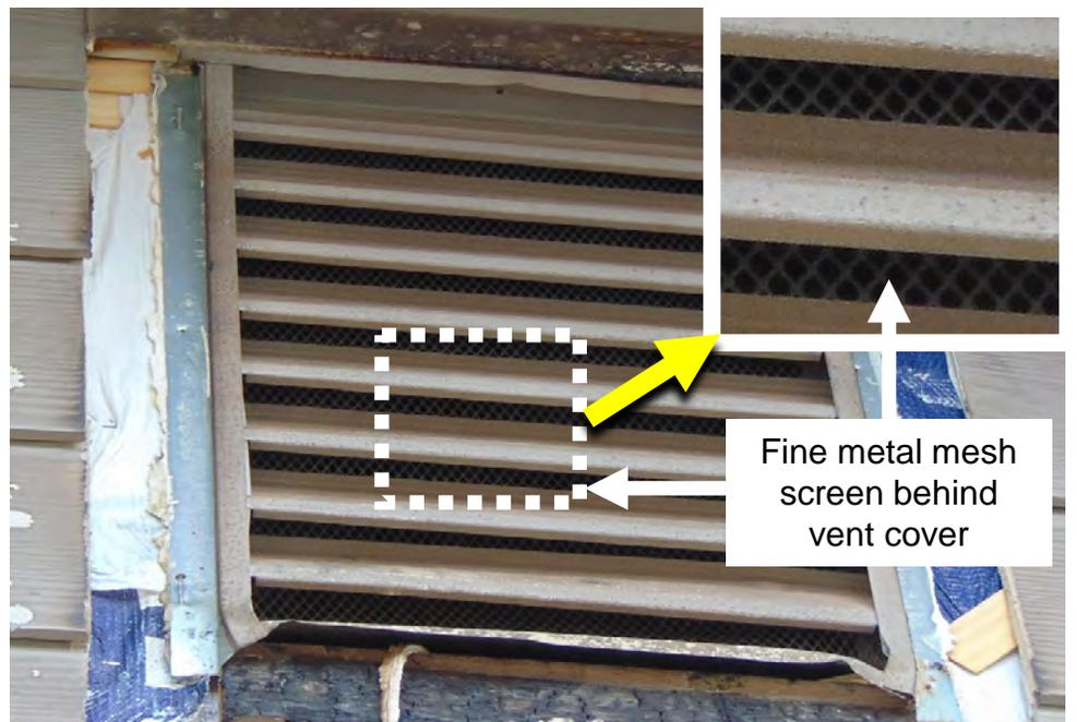
Item 13 Gable Vent – Apply 1/8<sup>th</sup> inch fine metal mesh screen inside gable vents to prevent ember intrusion.
