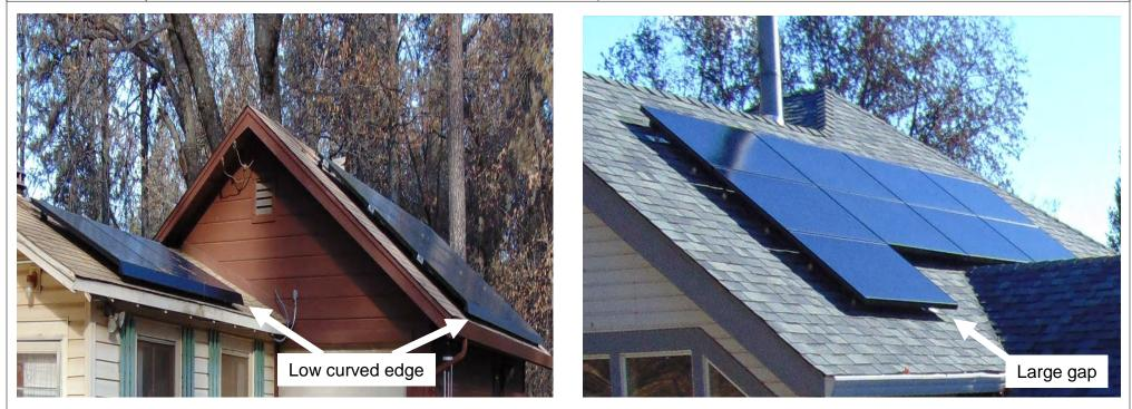
Item 4 Solar Panel Raised Up – Low curved edge can trap debris.
