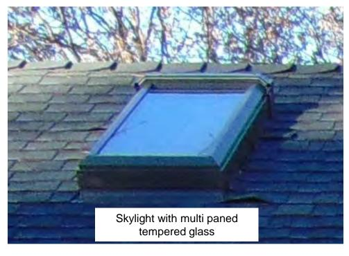
Item 1 Skylight – Skylights can melt or break from heat and allow ember intrusion.
